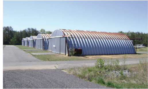
West Quonset Hanger, Facing SE
