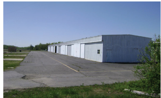
East Hanger, Facing SW
