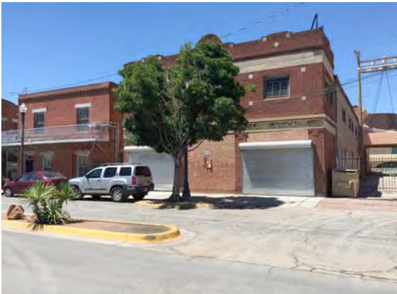
311 W. Overland (2 story warehouse), Alley
