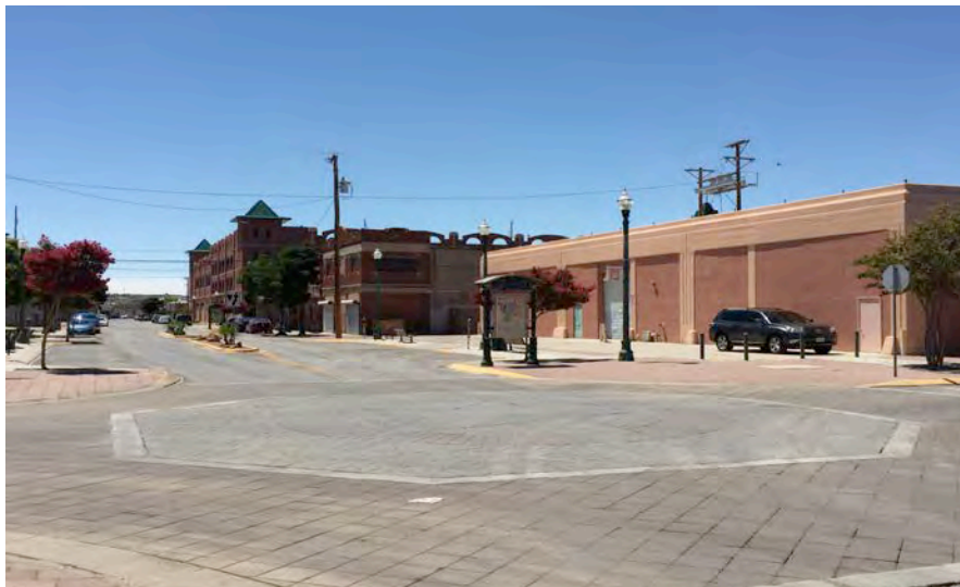
Sun Metro Parking/Transit Terminal + 315-317, 311, 301 W. Overland
