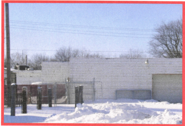
60 foot of rear warehouse entrance on South Morse.
