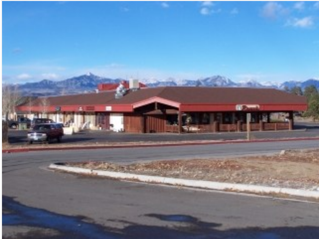
View from S/W Corner
