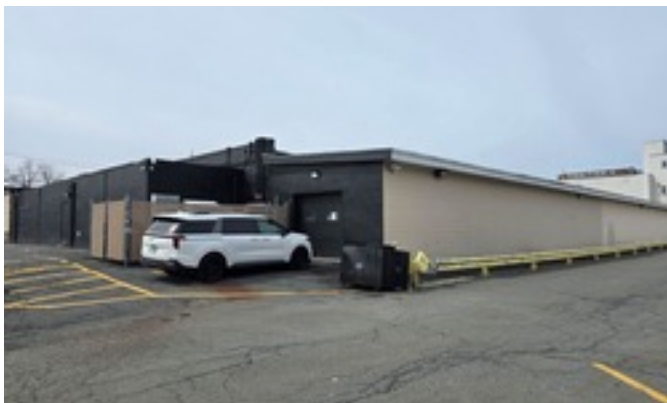
Loading and service access
