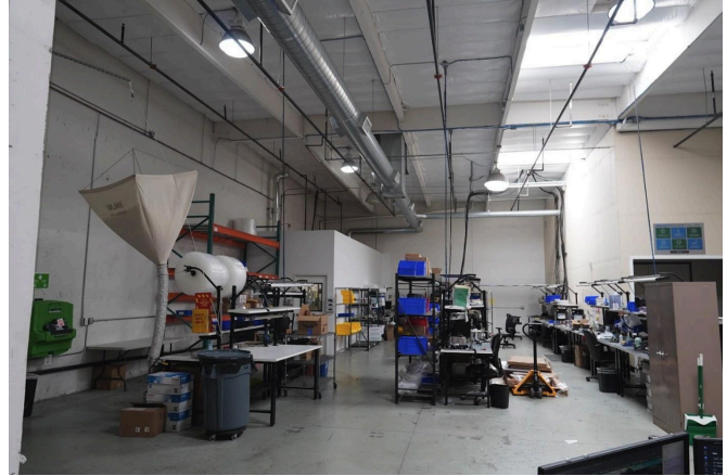
Warehouse — racking, HVAC, high clearance
