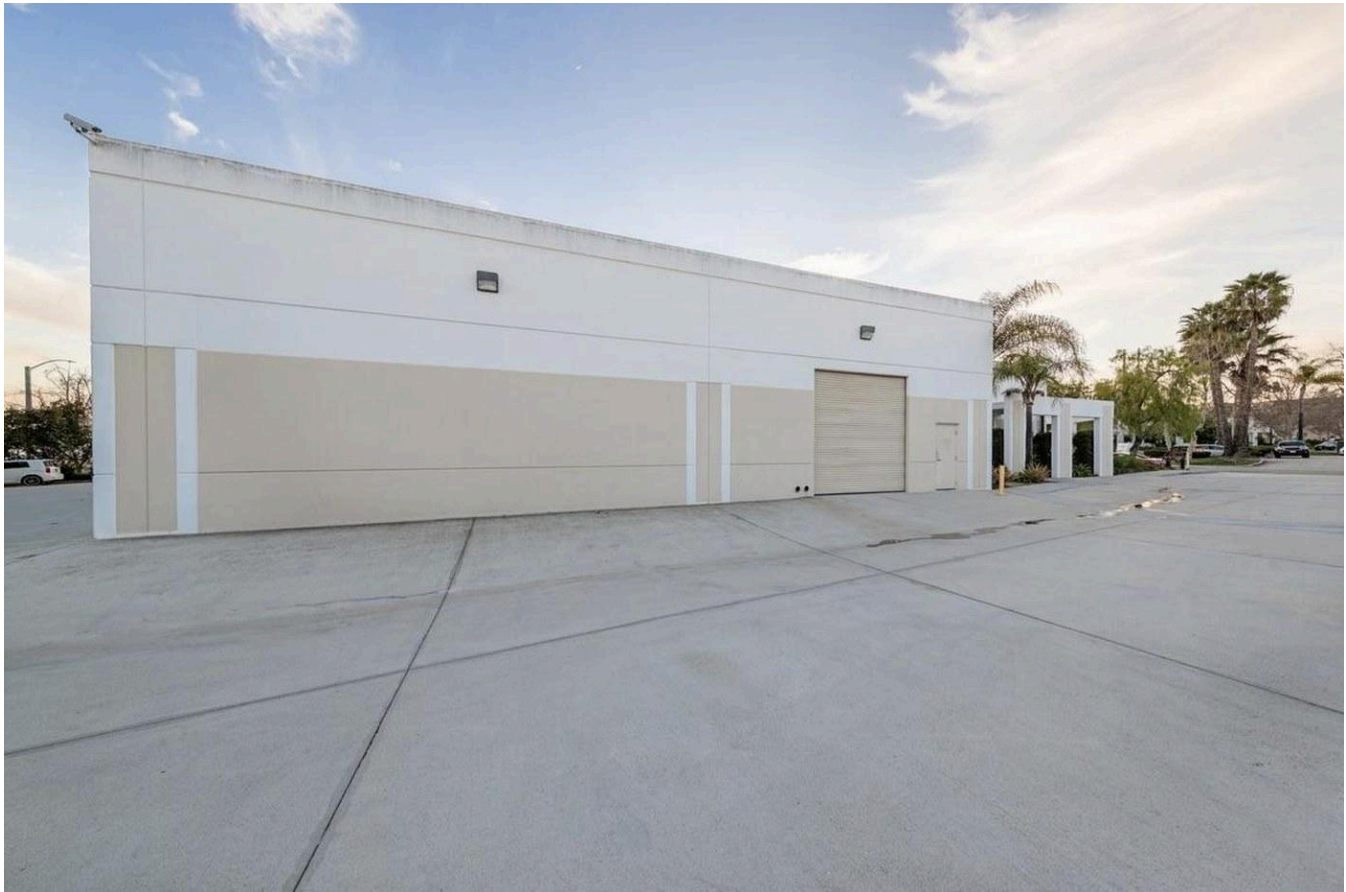
Drive-around concrete yard and grade-level loading
