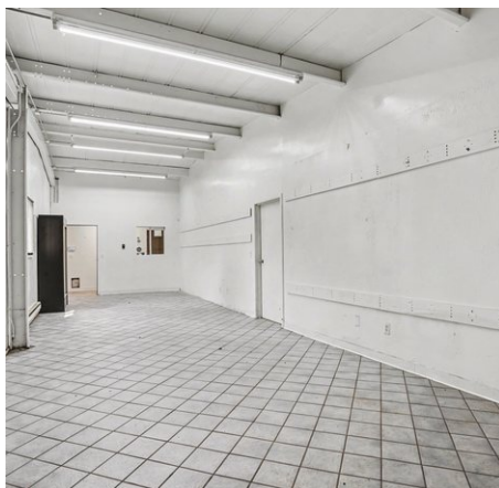
Finished front room — tile floor, service window
