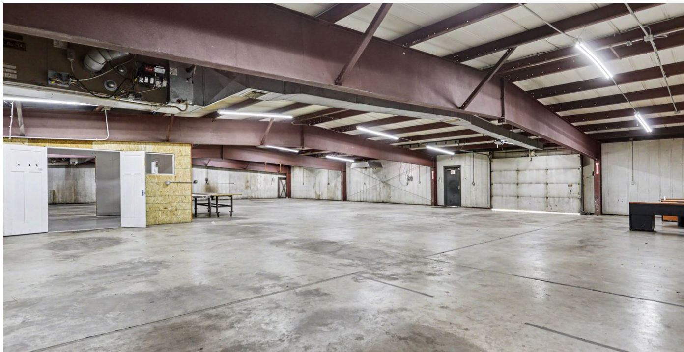
Clear-span shop — reinforced concrete slab, grade-level overhead door, three-phase 480V service, ducted heat and suspended linear lighting.
