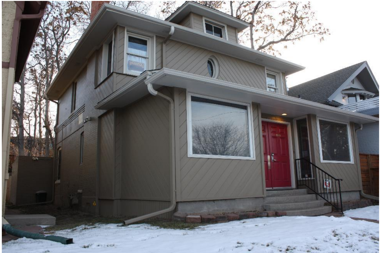
Front View of Building:
