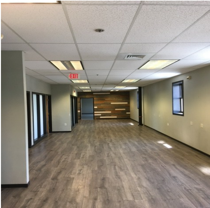
2,700 s.f. office section that is part of the 9,200 s.f. leased unit.
