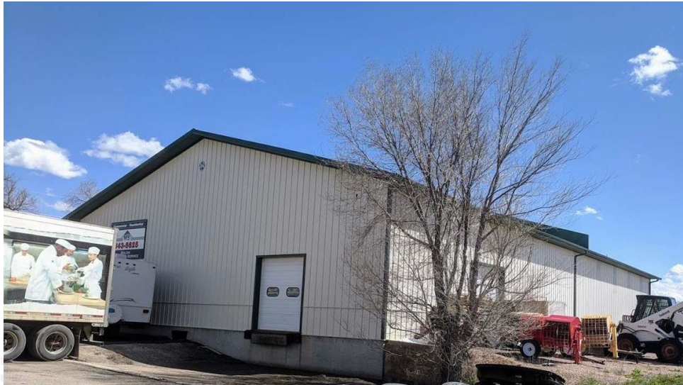
Two truck level loading docks
