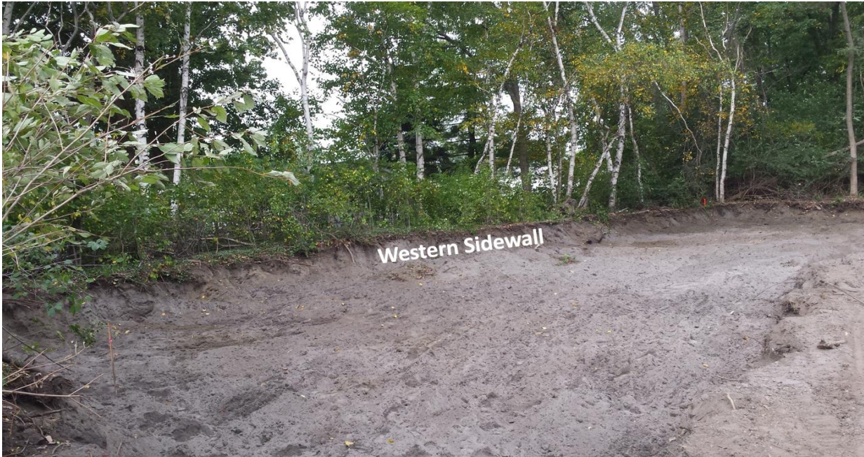
Image 4. Completed excavation, looking west.
