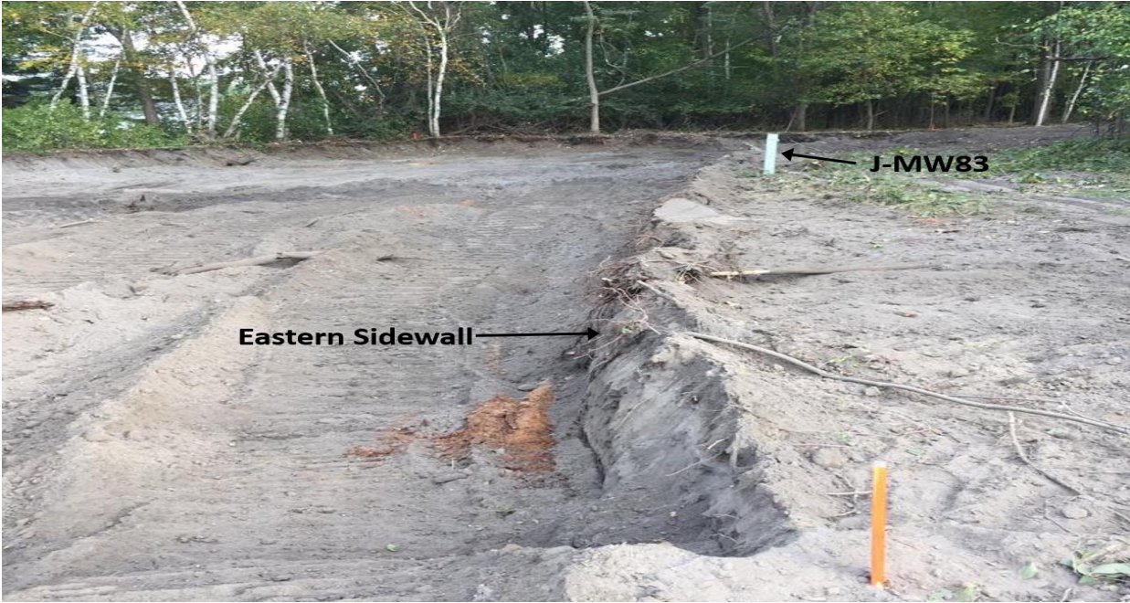
Image 6. Completed excavation, looking north.
