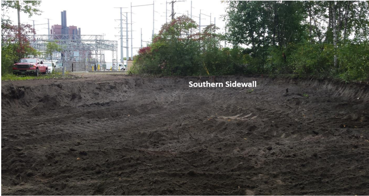
Image 3. Completed excavation, looking south.
