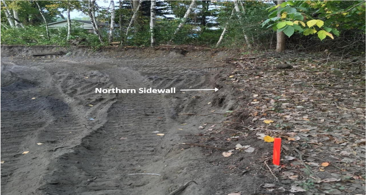
Image 5. Completed excavation, looking west.
