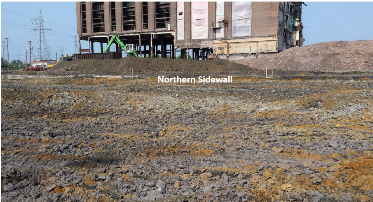
Image 6. Completed excavation, looking north.
