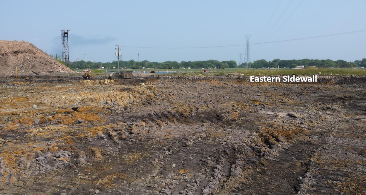
Image 3. Completed excavation, looking east.
