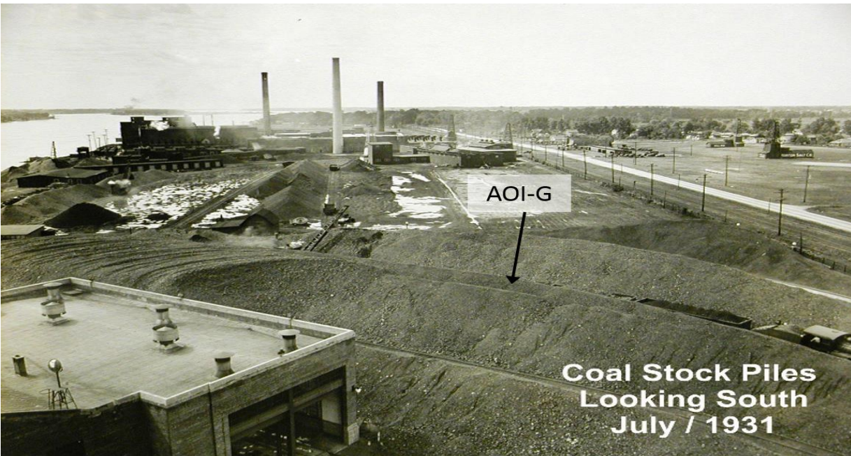
Image 2. Atop the MVPP building, looking south.
