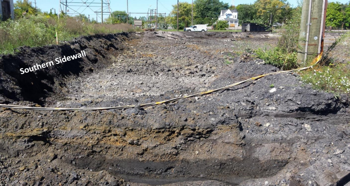
Image 4. Completed excavation, looking west.
