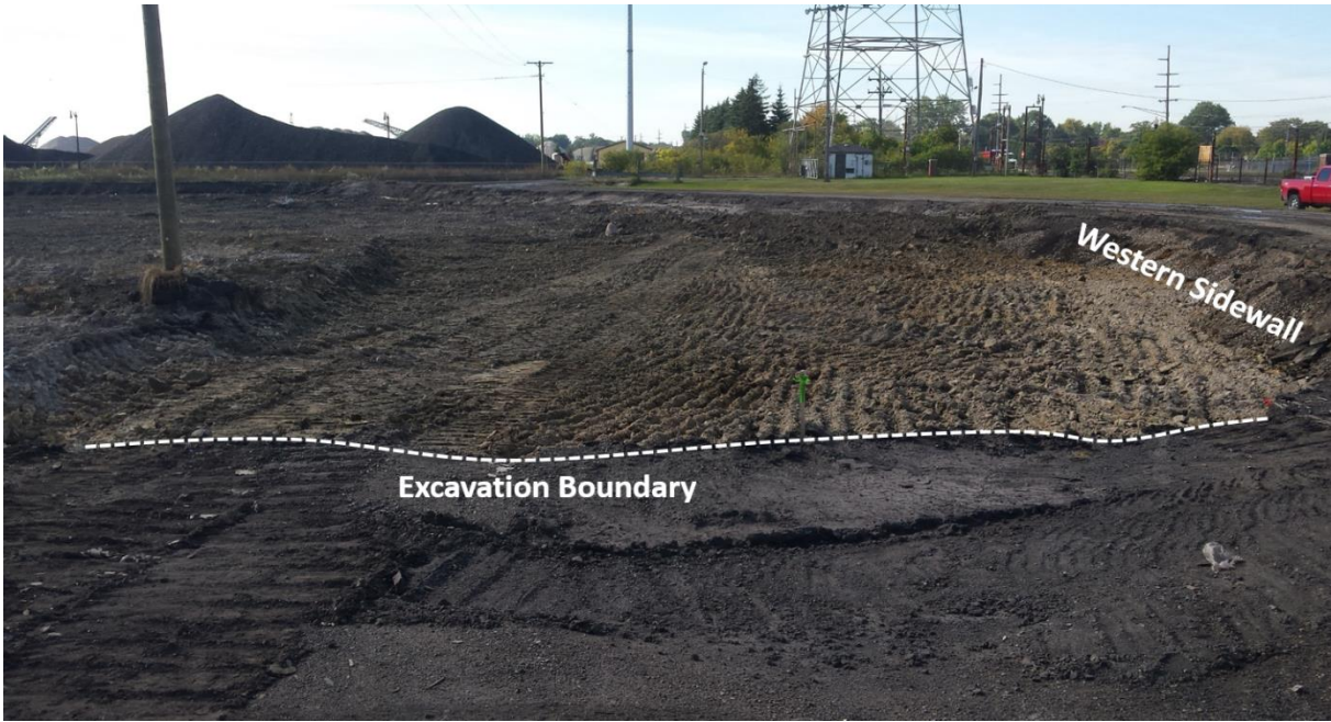
Image 5. Completed excavation, looking south.
