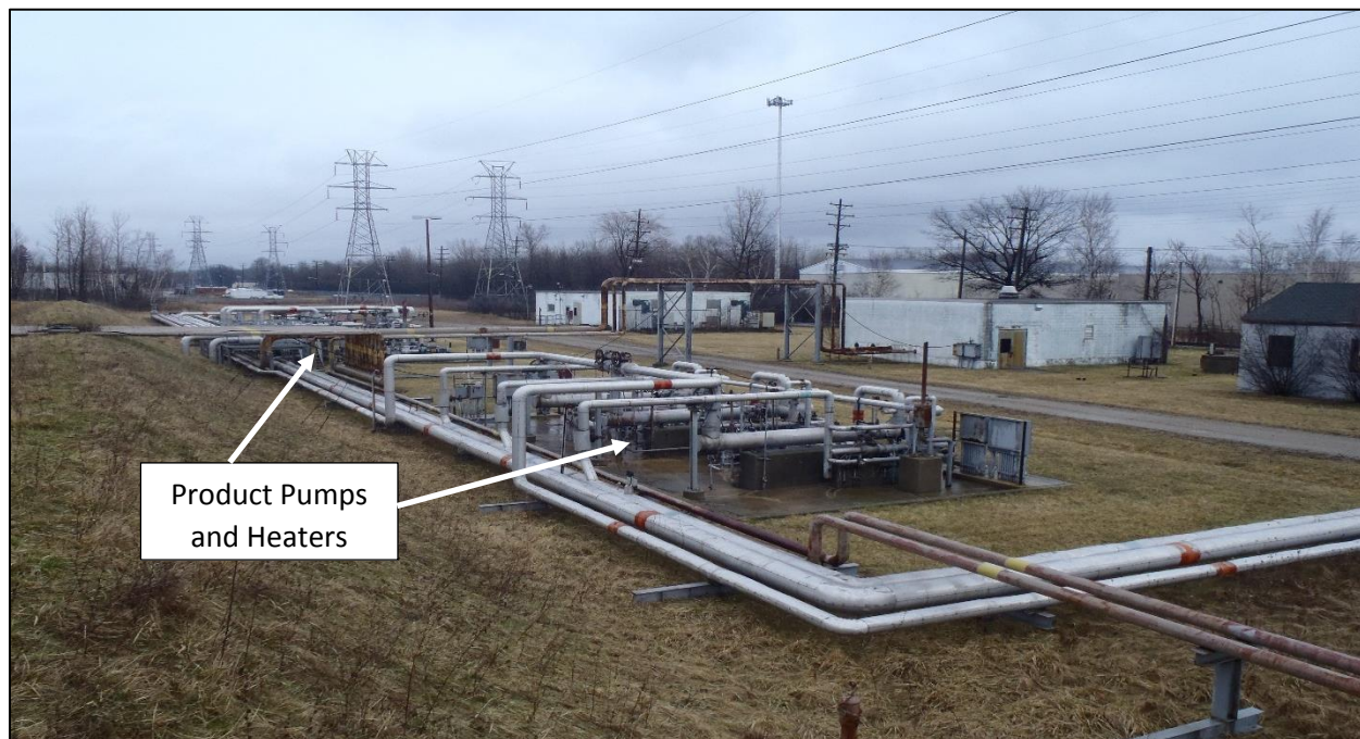
Image 2. Section of above ground piping, including product pumps and heaters. Looking north.
