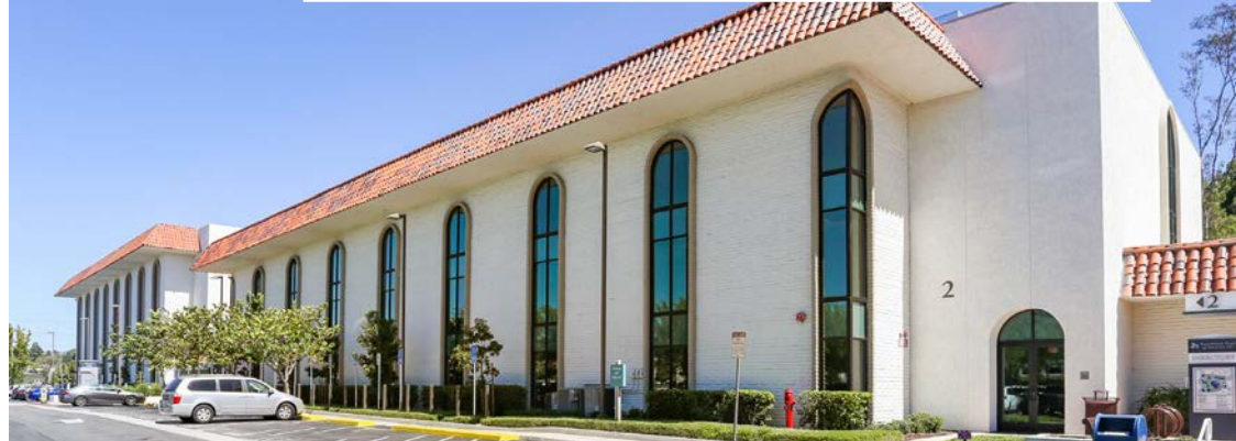
Medical Office Building II
