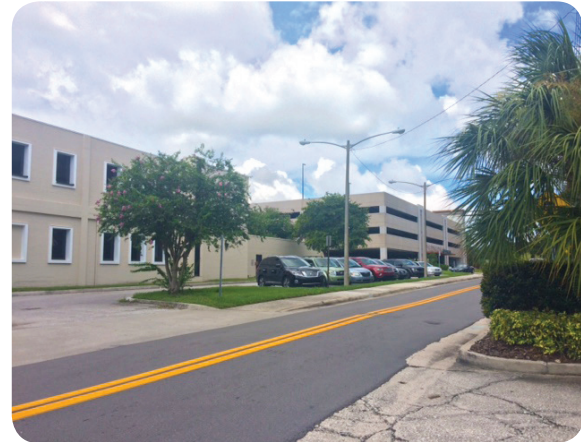
View towards County parking garage
