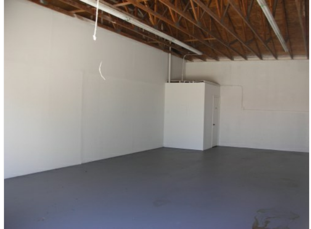
800 SF with Small Reception/Office 1290 E
