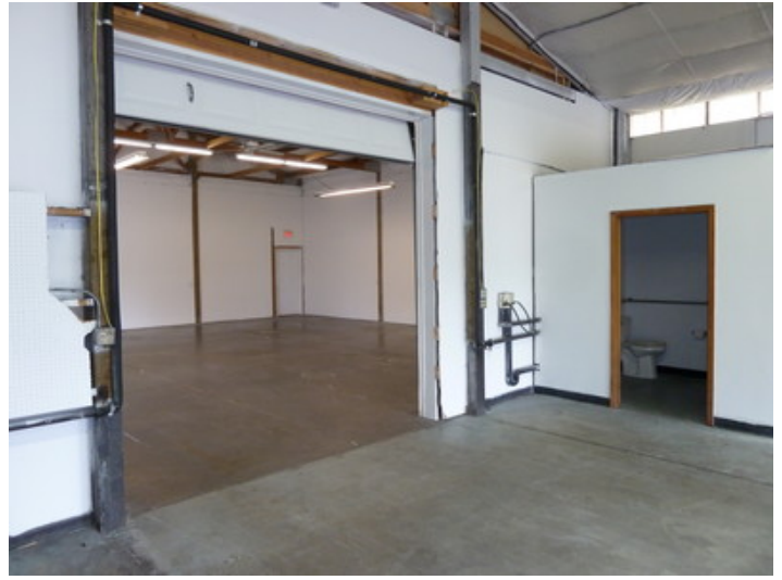
Rear bay door and restroom in front bay
