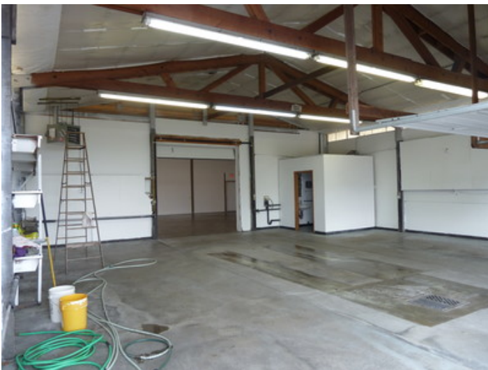
Front wash bay
